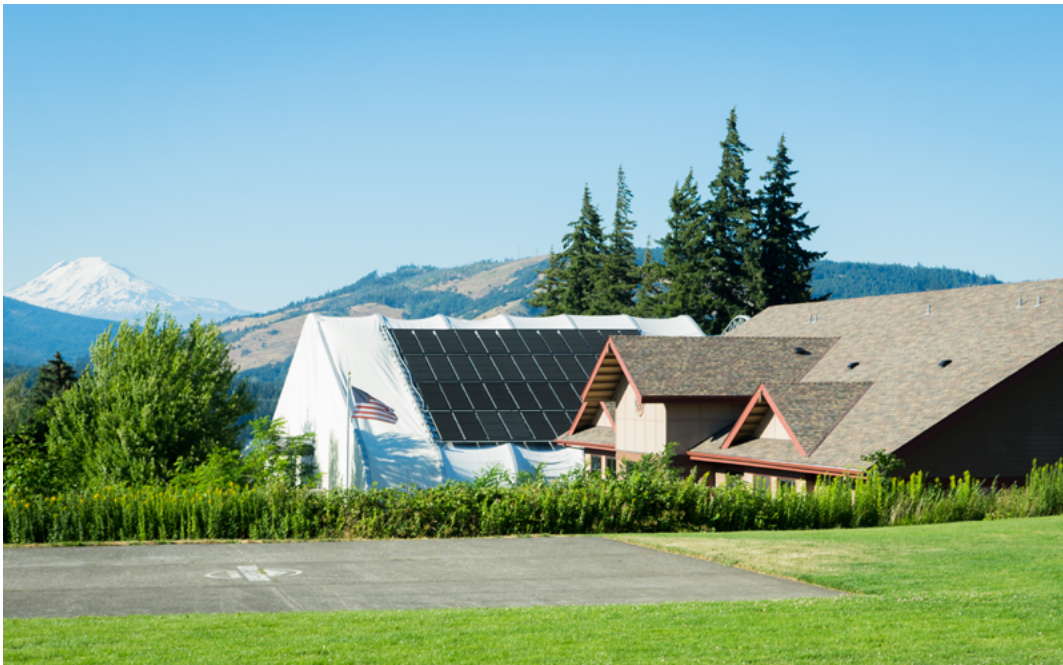
Solar panels on the Hood River Valley Aquatic Center, which were installed long before the energy plan. Legacy projects like this can provide great insight into community priorities. Photo credit: Lindsay McClure and Hood River Energy Council
