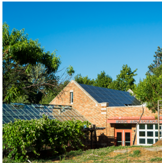
Solar panels on Hood River Middle School. Photo credit: Lindsay McClure and Hood River County Energy Council
