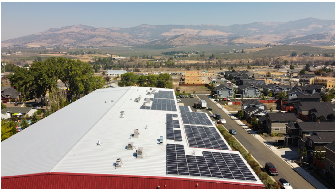
A Solarize Rouge solar array on the roof of the Oregon Shakeseare Festival’s production building in Talent. It includes both a community solar project and a project for OSF. Photo credit: Solarize Rogue and True South Solar
